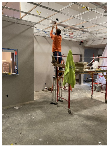
Installation of ceiling grid in Administration work area
